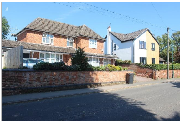
Figure 2-12 Boundary walls on Main Street
