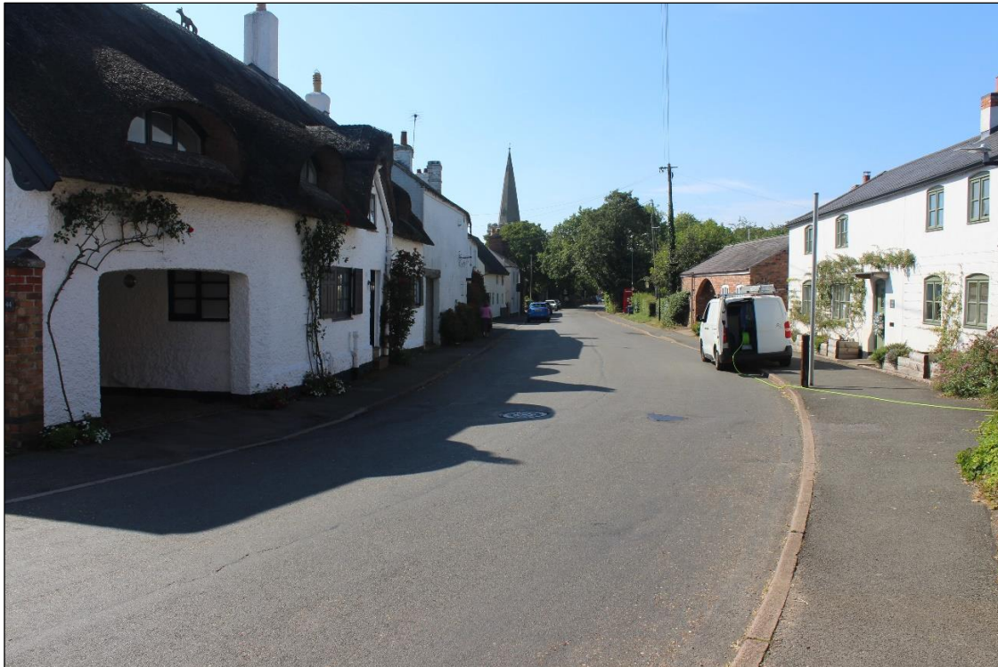
Figure 2-8 View south down Main Street towards St Catharine's Church
