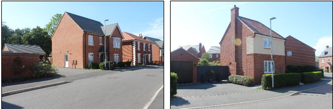
Figure 2-14 Unattractive plain slab wall contrasting with brickwork details providing a more attractive view from the street.
