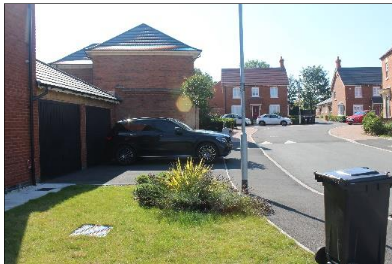
Figure 2-16 Insufficient setback in new development
